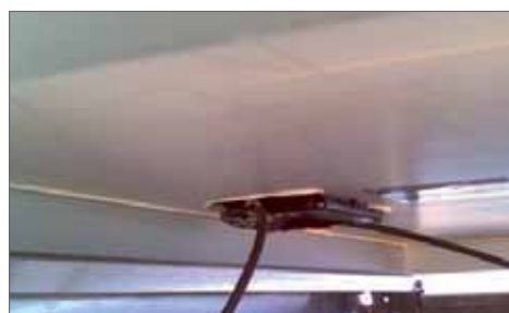
The FLIR T335 thermal imaging camera can also be used to scan the other components of the solar installation, such as this faulty connector.
